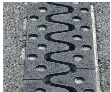
mageba RSFD cantilever finger joint with ROBO®GRIP
