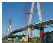
Can Tho Bridge (VN)
