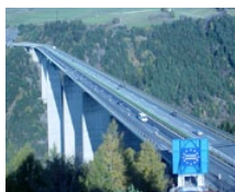
Europe Bridge (AT)
