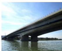
Traismauer Bridge (AT)
