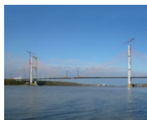
Audubon Bridge (USA)
