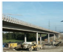
Wasserbachtal Bridge (DE)
