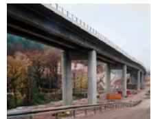
Mönchröden Bridge (DE)
