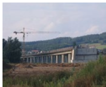
Maintal Bridge (DE)
