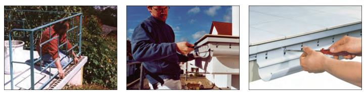
The Schluter®-BARA edging profiles and Schluter®-BARIN gutter system finish and protect the edges of the assembly and provide water management at balcony and terrace perimeters.
