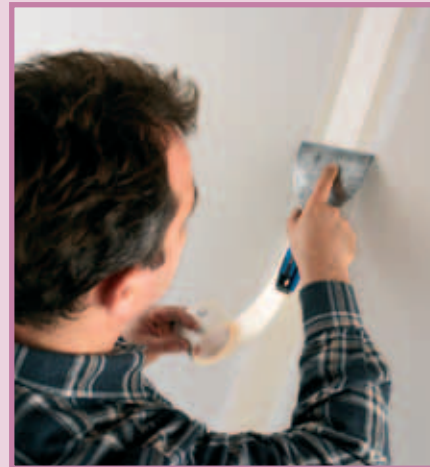
Prepare the wall
